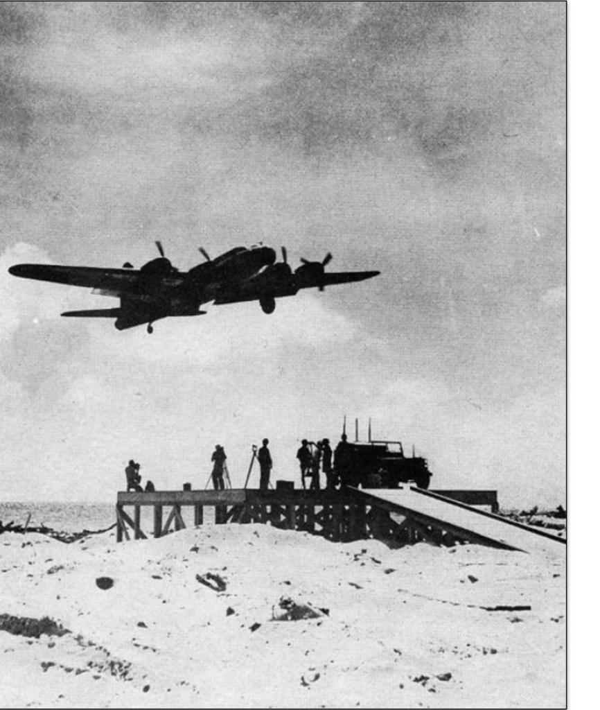
A B-17 drone, controlled by transmitters on the ground, lands at Eniwetok during Operation Crossroads in the Marshall Islands.
